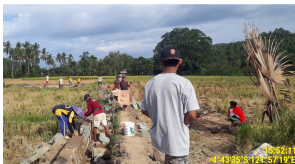
Picture 4. Irrigation channel works
