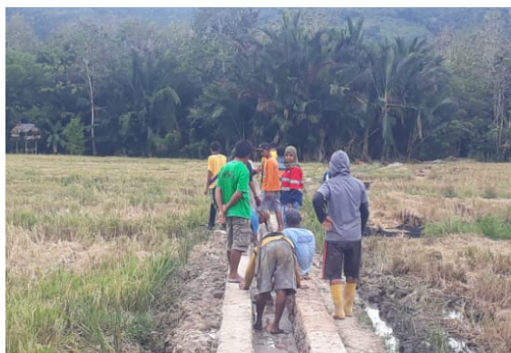
Picture 3. Assistance in Building Irrigation Canals
